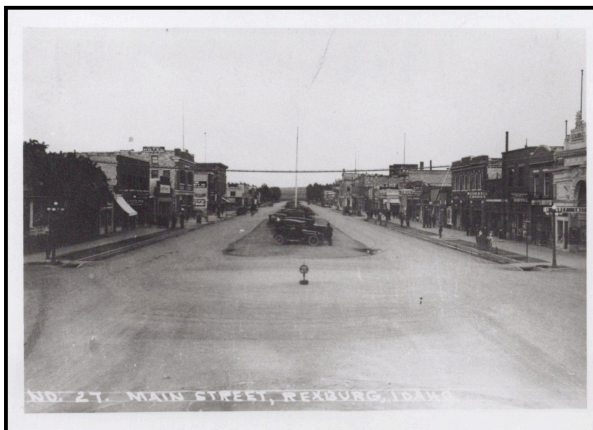
Main Street looking east with an island down the middle.
